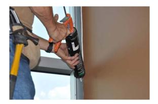
D. Apply a continuous bead of acoustical sealant between the unexposed 3/4" blanket edge and the vertical drywall edge of the partition wall.
